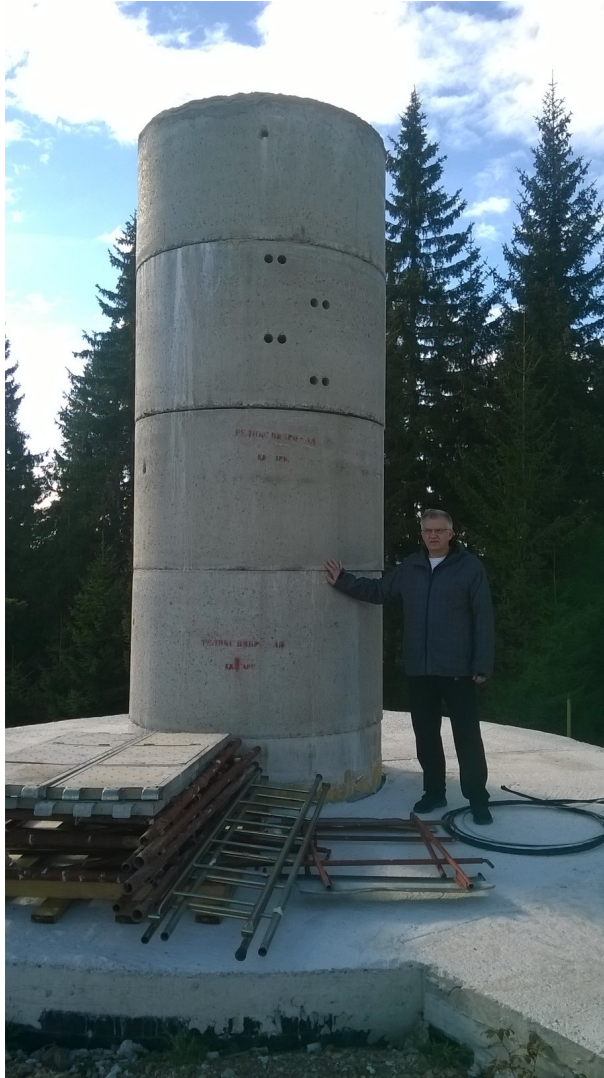
Figure 2: The concrete pillar of new 1.5 m telescope (in November 2022) at Rozhen NAO BAN (Bulgaria).
